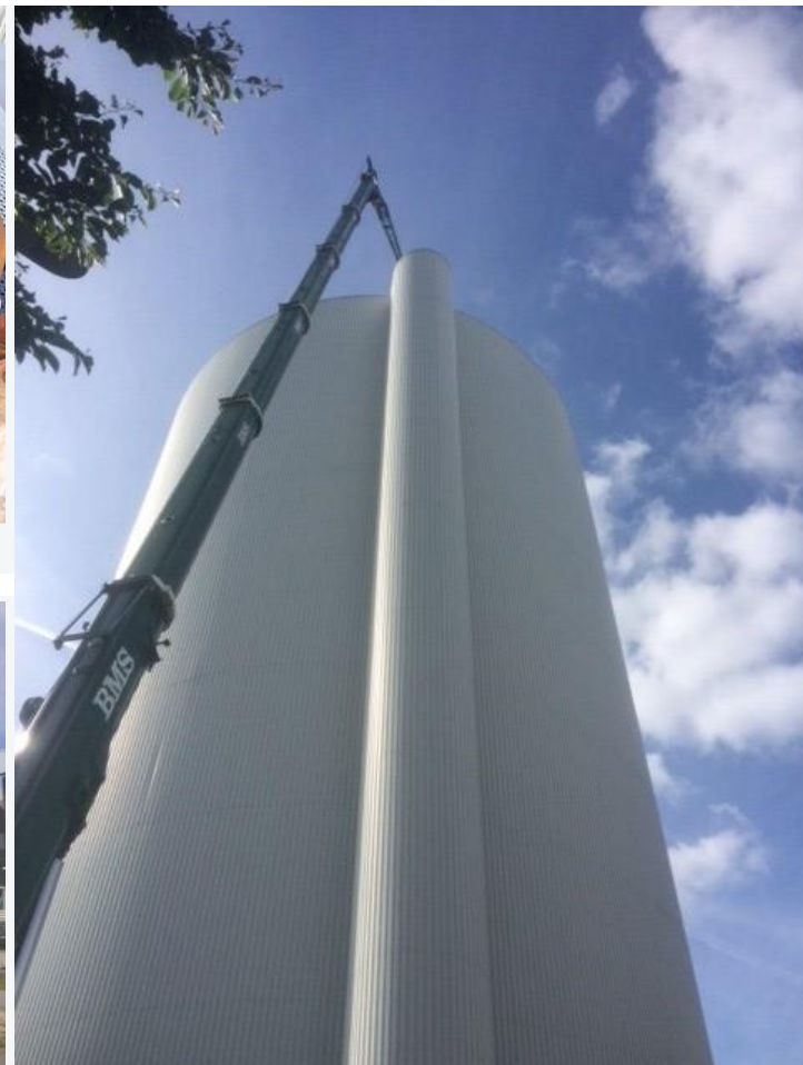
BMS crane for lifting the ROV to top of storage tank
