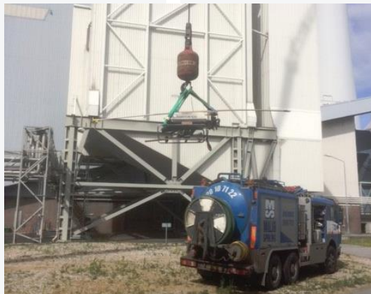
Sludge exhauster for extraction of sediment samples
